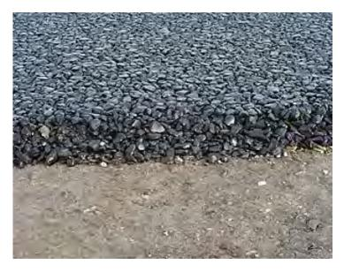
The asphalt is 25 years old, surpassing the useful life of 20 years. The condition is less than average and the sealcoating project in 2013 just masked the condition.
