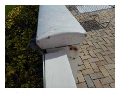
An aluminum fence can last for a very long time. Upon inspection we found the fence in average condition with a peeling surface. Replacing the fence will be foremost a cosmetic decision. We estimate a useful life of 30-35 years.
